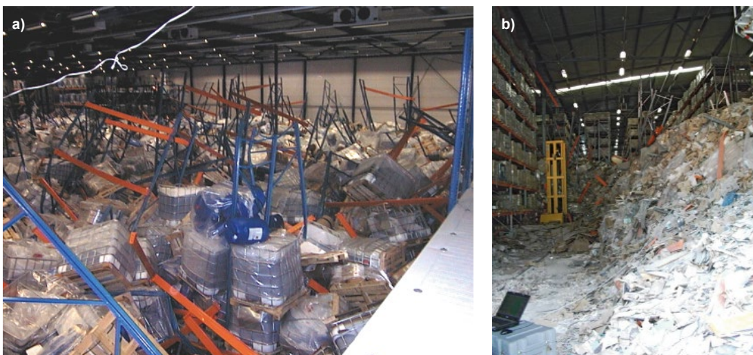
Fig. 33. a) A minor collision can result in total collapse due to the dynamics of pallets falling; b) in many cases lift trucks are involved in collapses
